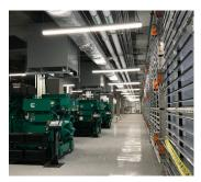
The electrical distribution system design is primarily focused around concurrent maintainability, i.e., maintaining power delivery paths to the customer during maintenance activities. "We are running paralleled generators — what we call the ring bus — divided into two generator segments. We always maintain adequate gens in case a section ever needs to be taken down
